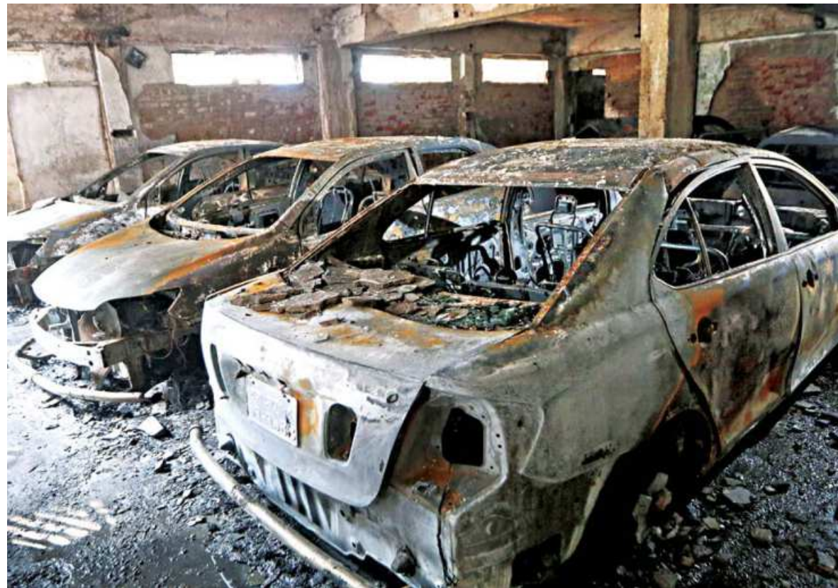
Charred remains of parked cars inside a building on Dilu Road in the capital's Eskaton. A devastating fire in the building yesterday morning left three people dead and two others critically injured.
