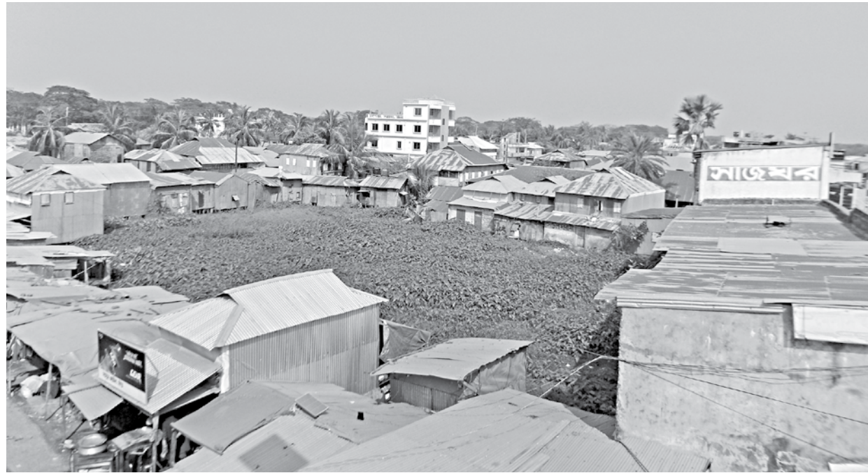
One of the three government ponds, in Mohipur Bazar of Patuakhali's Kalapara upazila, that the encroachers have put on death throes by building structures on its land and dumping waste in it.
