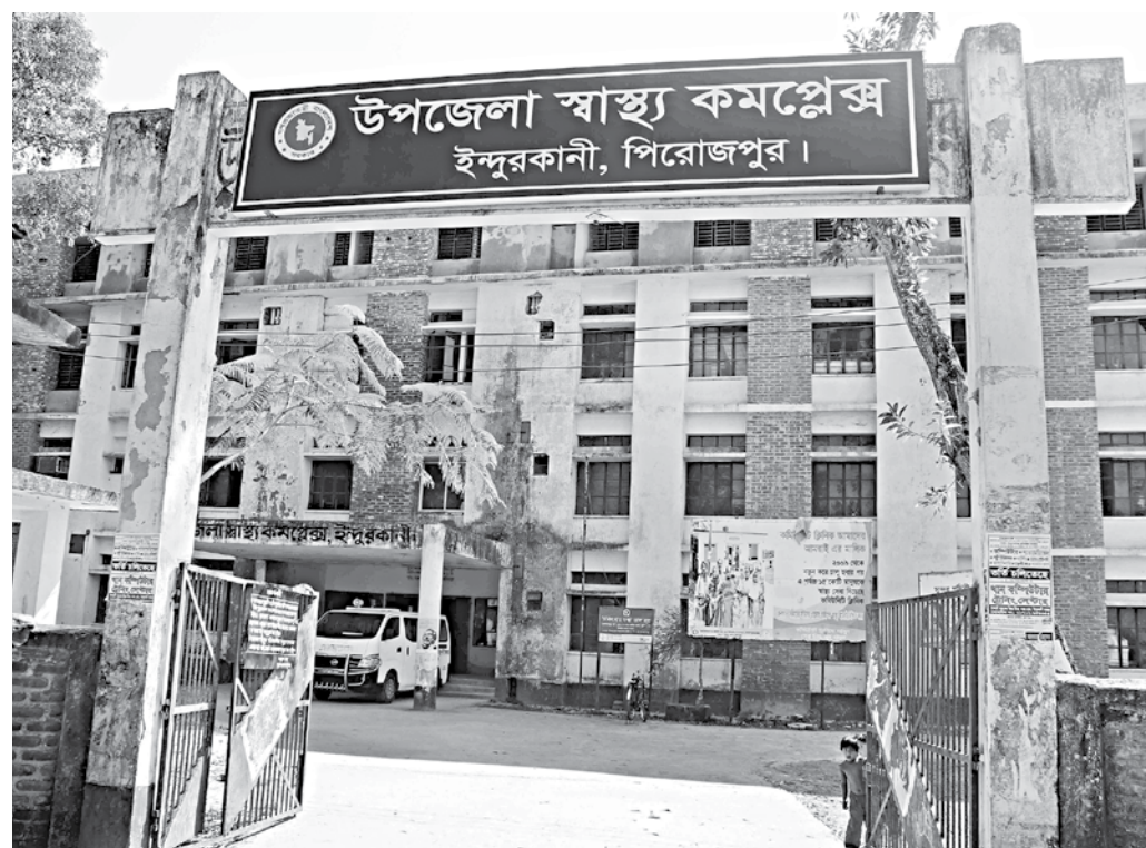
Indurkani Upazila Health Complex in Pirojpur.
