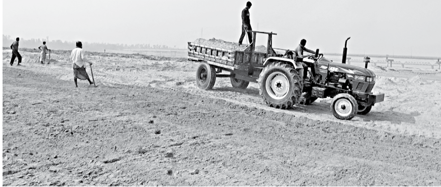
Mindless sand lifting from Teesta riverbed at Teesta village in Lalmonirhat Sadar upazila poses erosion threat to nearby Teesta Road Bridge.
