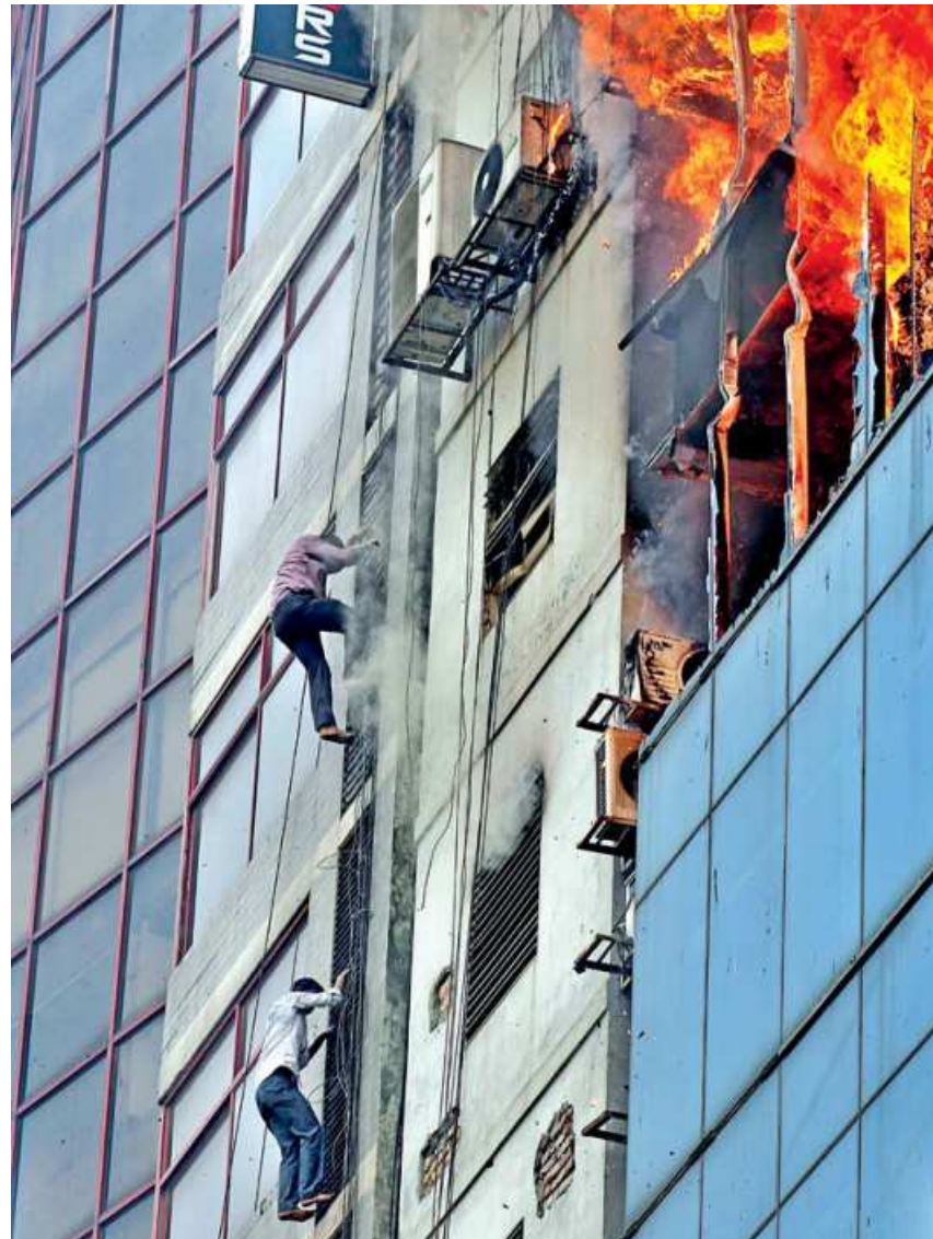
Fire outbreak at FR Tower in Banani on March 28, 2019.
