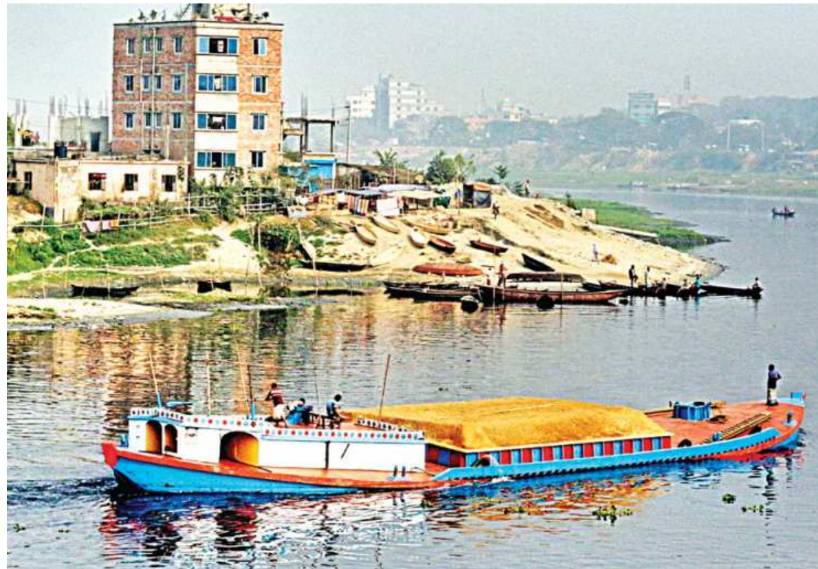
Several structures, including a four-storey building, have been set up on the Turag as grabbers occupy a large part of the river near the BIWTA landing station at Sinnirtek in the capital's Mirpur area. With the authorities carrying out occasional eviction drives, such encroachment on the river land has been going on for years. The photo was taken on Thursday.
