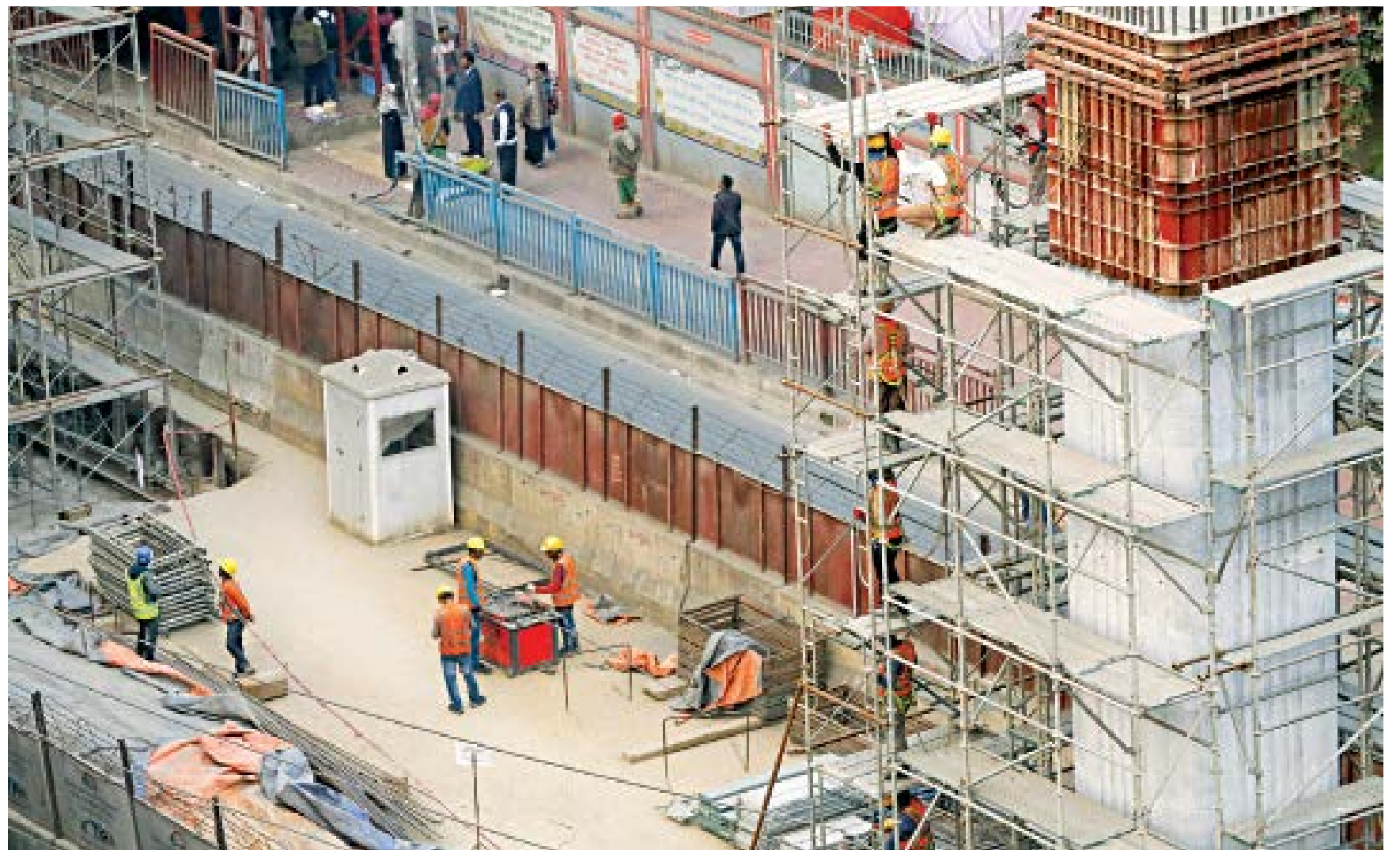
Labourers at work at the CP-05, MRT Project site.
