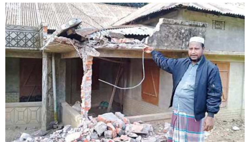
A man stands beside his house near the Dhamai river in Moulvibazar's Barlekha upazila. A portion of the house has been demolished in an eviction drive recently.
