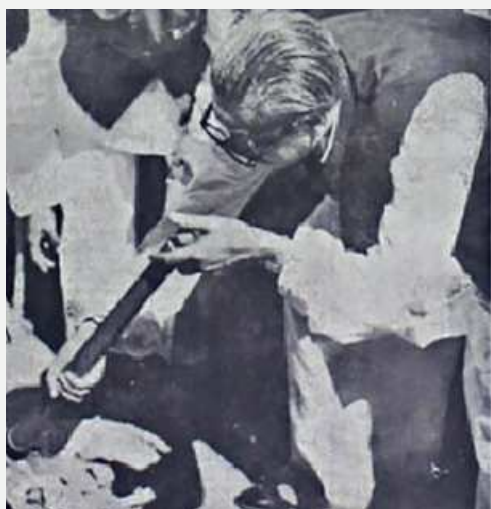
Bangabandhu is seen excavating soil with a spade in the WAPDA embankment at Ramgati, Noakhali on February 20, 1972.
