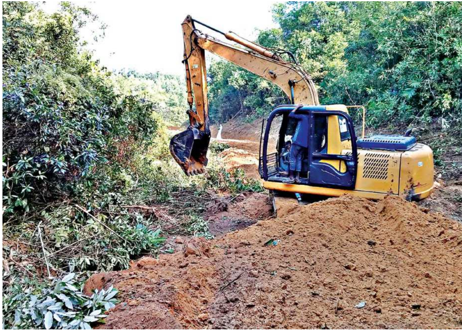
Defying a court order, an excavator, deployed by Halda Valley, clears trees at a hillock at Ramgor-Sitakunda forest in Chattogram's Fatikchhari upazila to make a road. The photo was taken last month.
