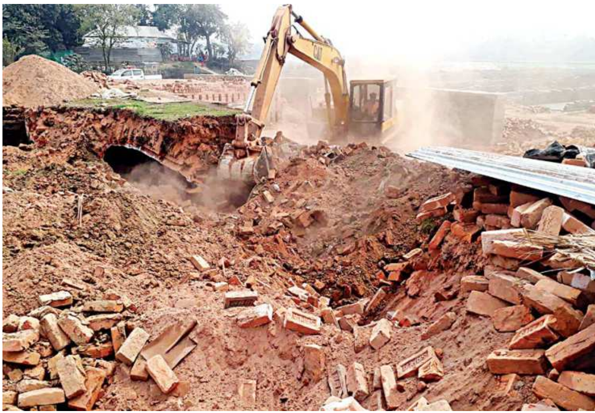
A bulldozer destroying bricks at an illegal brick kiln in Gazipur city's Dhitpur area on Monday. Department of Environment conducted a mobile court drive there. Toxic fumes emitted from brick kilns are largely blamed for the poor air quality in and around the capital.
