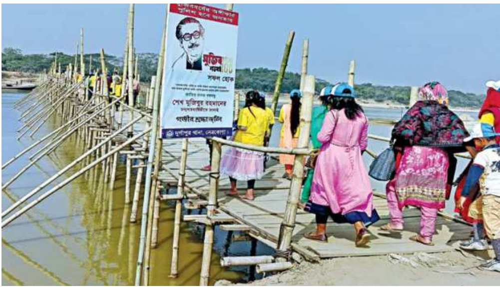
The newly built wooden bridge on the Sumeshwari river finally brings relief to people of 100 villages in Netrakona's Durgapur upazila.
