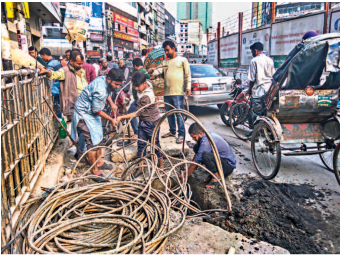
With the metro rail construction taking up around 60 percent of the road, maintenance work of fibre optic cables is eating up precious space on a street in Purana Paltan. Not only this, the work is also being done unsafely, with unprotected cables being piled by the side and no safety signs in sight.
