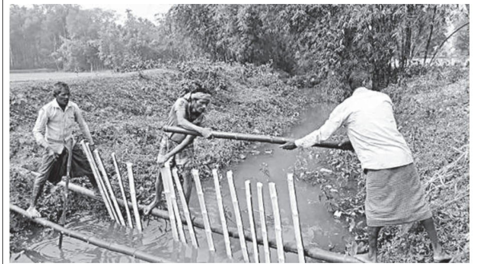
In their attempt to retain water for irrigation, locals building a makeshift dam with bamboo in Baliachhara canal near Kamalganj upazila headquarters in Moulvibazar. The photo was taken recently.
