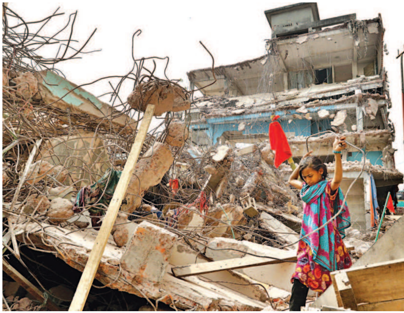
A girl walks on the rubble of a five-storey building, illegally built on the Turag river, after a part of the structure was knocked down by Bangladesh Inland Water Transport Authority during an eviction drive in Tongi's Abdullahpur area yesterday.
