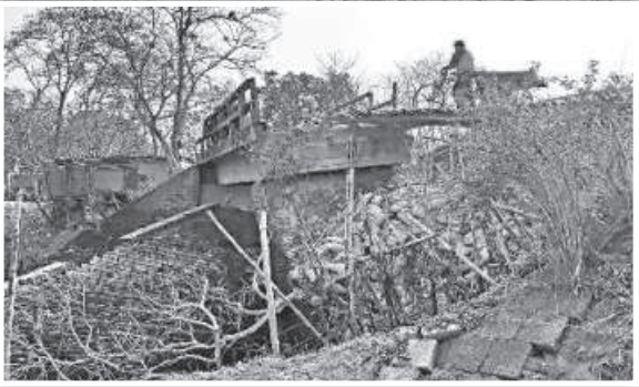
The span of the damaged bridge, on Panaullah canal in Boktarpur area of Natore's Singra upazila, lies precariously on top of its broken pier. Inset, a man pulls a rickshaw-van on the bamboo platform that the locals made to be able to use the bridge.
