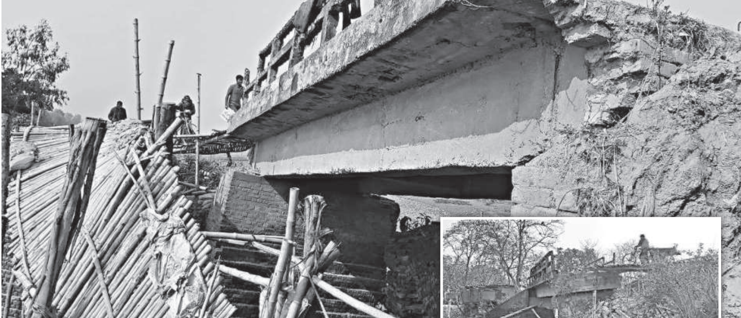
The span of the damaged bridge, on Panaullah canal in Boktarpur area of Natore's Singra upazila, lies precariously on top of its broken pier. Inset, a man pulls a rickshaw-van on the bamboo platform that the locals made to be able to use the bridge.
