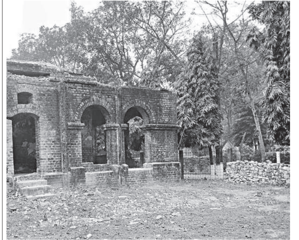
Without any arrangement of regular guarding, bricks removed from the proposed archaeological site of 175-year-old 'nilkuthi' at Notkhana village in Polashbari union of Nilphamari Sadar upazila lie in front of the historic structure on Sunday. The district police, who employed labourers to break the structure on December 24 last year, stopped the work shortly after serious objection by locals.
