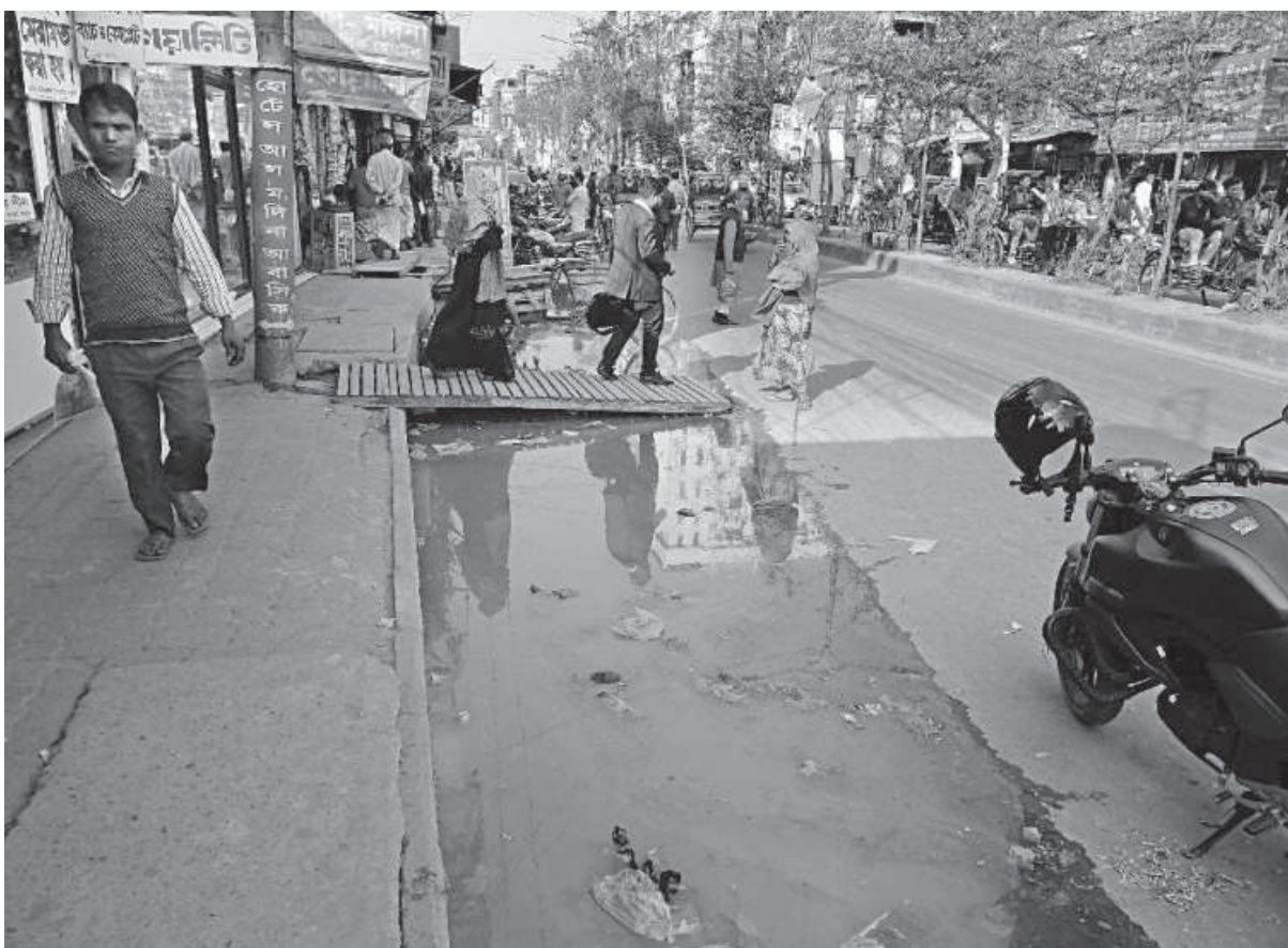
Sewage from an overflowing drain covers part of this road in Satmatha intersection area of Bogura town. The photo taken yesterday gives a typical picture of the awful drainage system in the important area under the municipality, thanks to the callousness of the authorities concerned.
