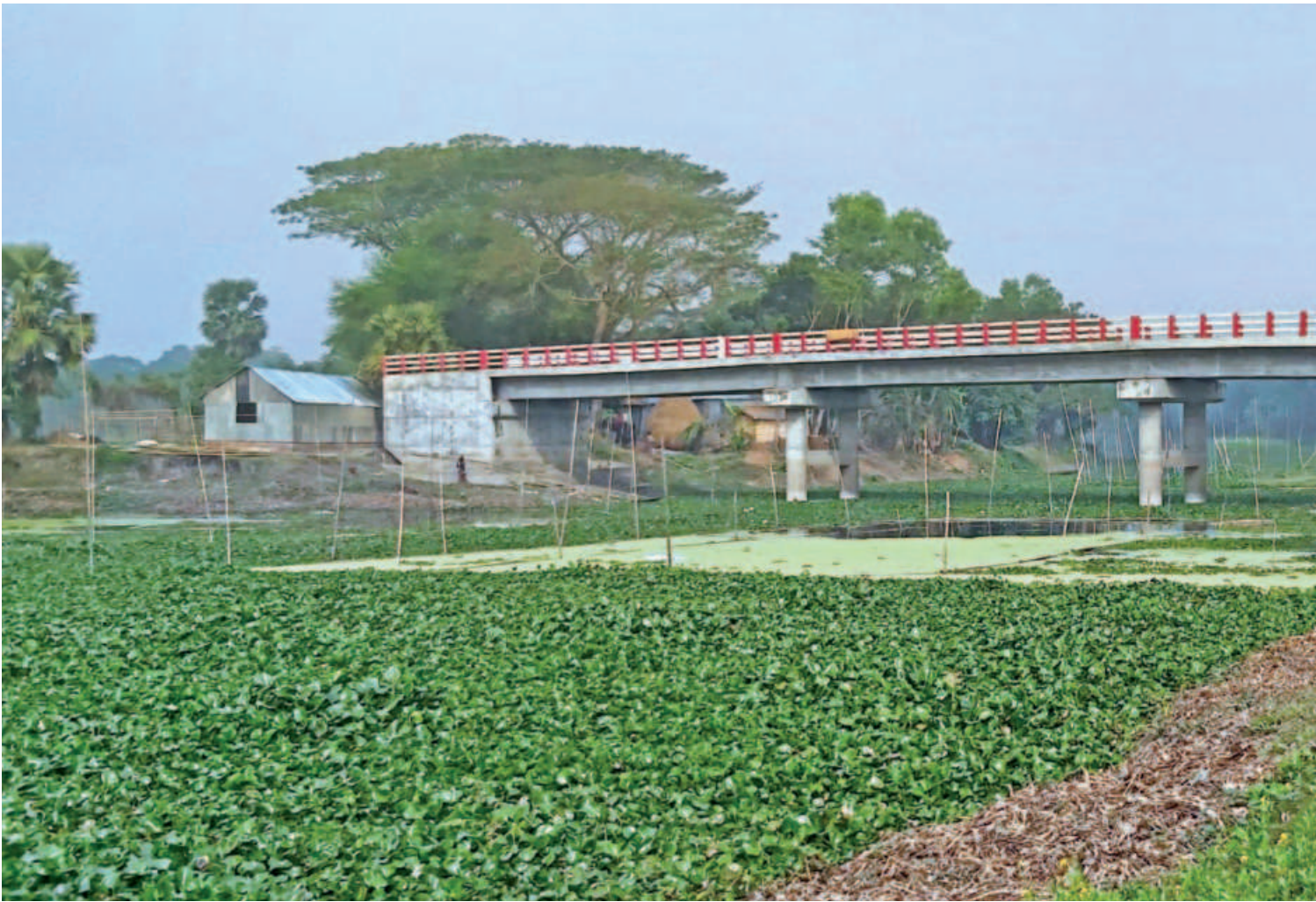
This 60-foot-long bridge over a canal in Kamlapur area of Gopalganj’s Musksudpur upazila is of no use as there is no approach road on one side of the structure. The bridge was built by the Local Government Engineering Department nearly two years ago. The photo was taken recently.
