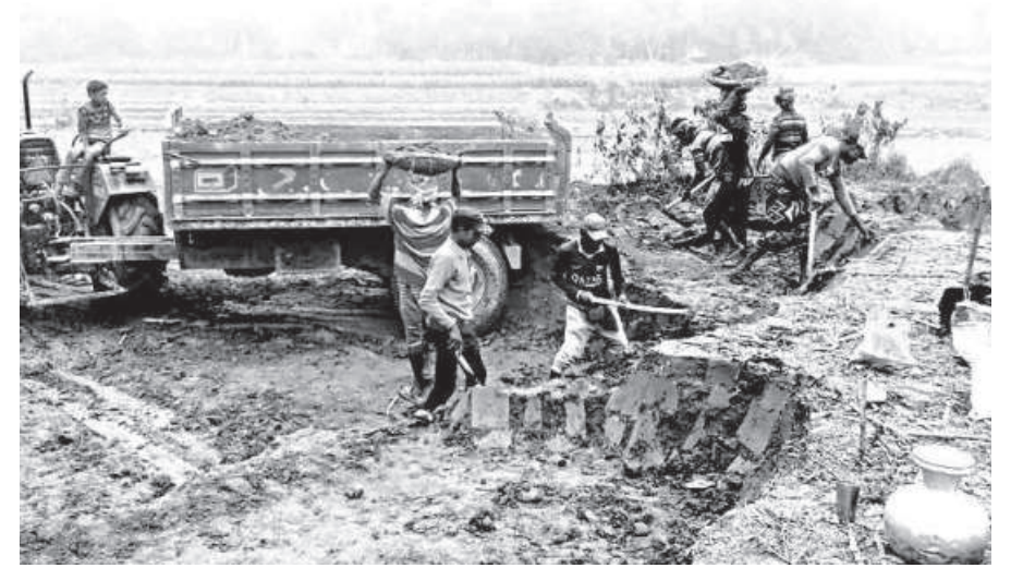
Workers loading up a tractor wagon with earth illegally cut from the bank of the Bhairab river in Mahajanpur village of Meherpur's Mujibnagar upazila. The photo was taken recently.
