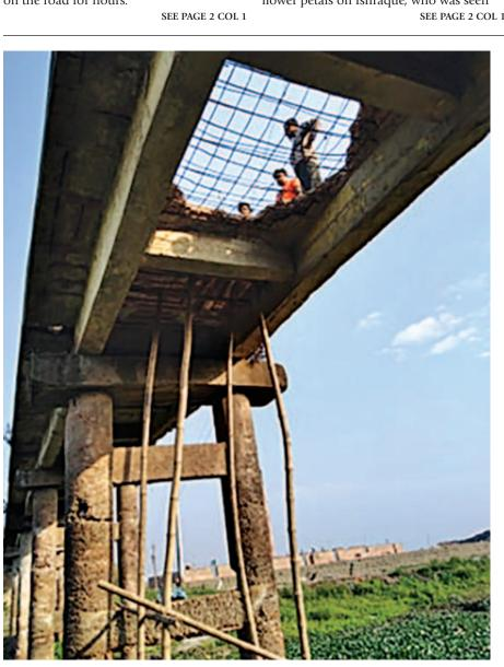
People looking down a hole on the bridge in Gabtola area of Brahmanbaria town after a large chunk of concrete fell off last week. Local autorickshaw pullers have placed bamboos in an effort to make the rickety bridge steady. The hole was eventually patched up with a slab of metal.
