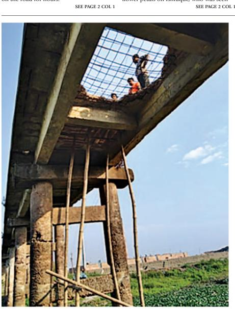
People looking down a hole on the bridge in Gabtola area of Brahmanbaria town after a large chunk of concrete fell off last week. Local autorickshaw pullers have placed bamboos in an effort to make the rickety bridge steady. The hole was eventually patched up with a slab of metal.
