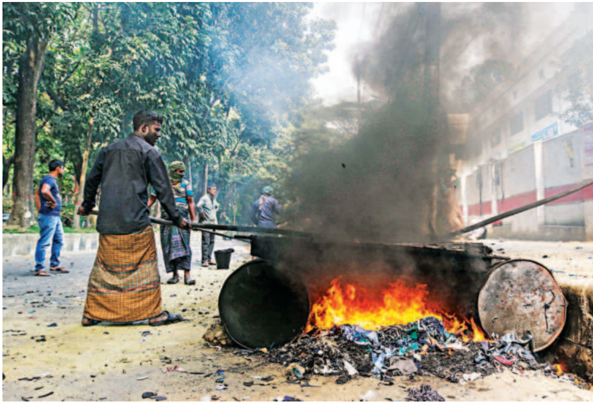
A thick cloud of smoke billows from a makeshift burner in front of Chattogram's Bangladesh Railway Hospital yesterday. To repair roads, labourers are burning scrap from RMG factories to melt bitumen. At a time when environmental concerns are at a peak, reckless actions like this are putting both the nature and people at risk.
