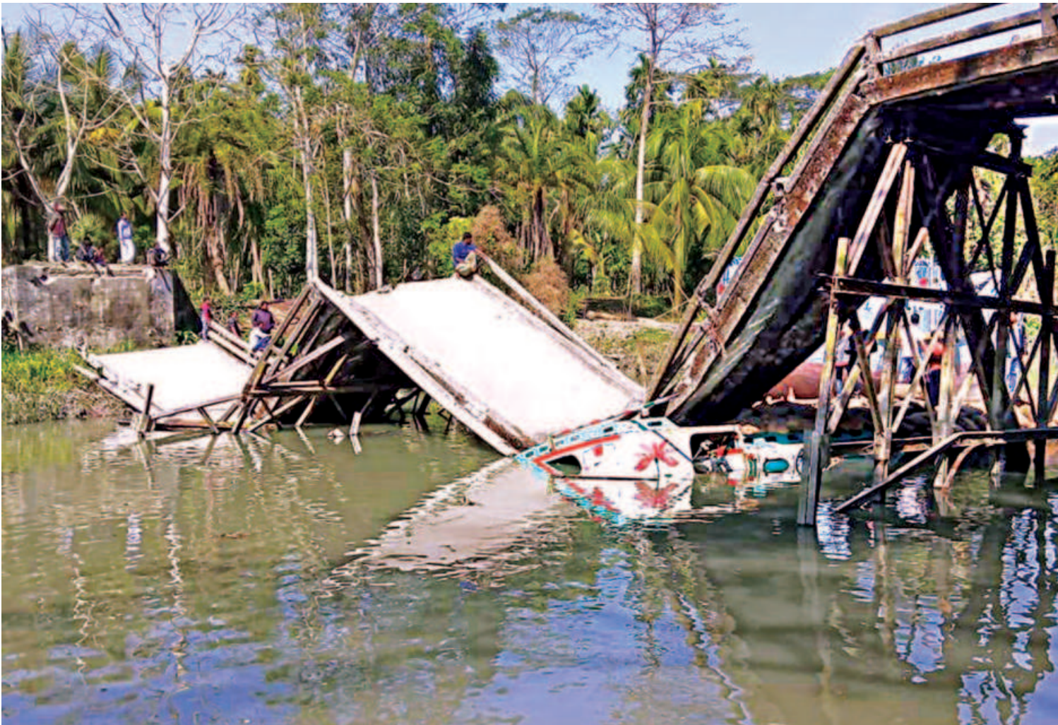
A sinking paddy-laden trawler that hit an iron bridge, causing it to collapse, in Domrabad-Hosnabad area of Patuakhali's Mirzaganj upazila on Tuesday. The accident has caused disruption to road communications between Patuakhali's Mirzaganj and Barguna's Betagi upazila and waterways communications between Jhalakathi and Khulna districts.
