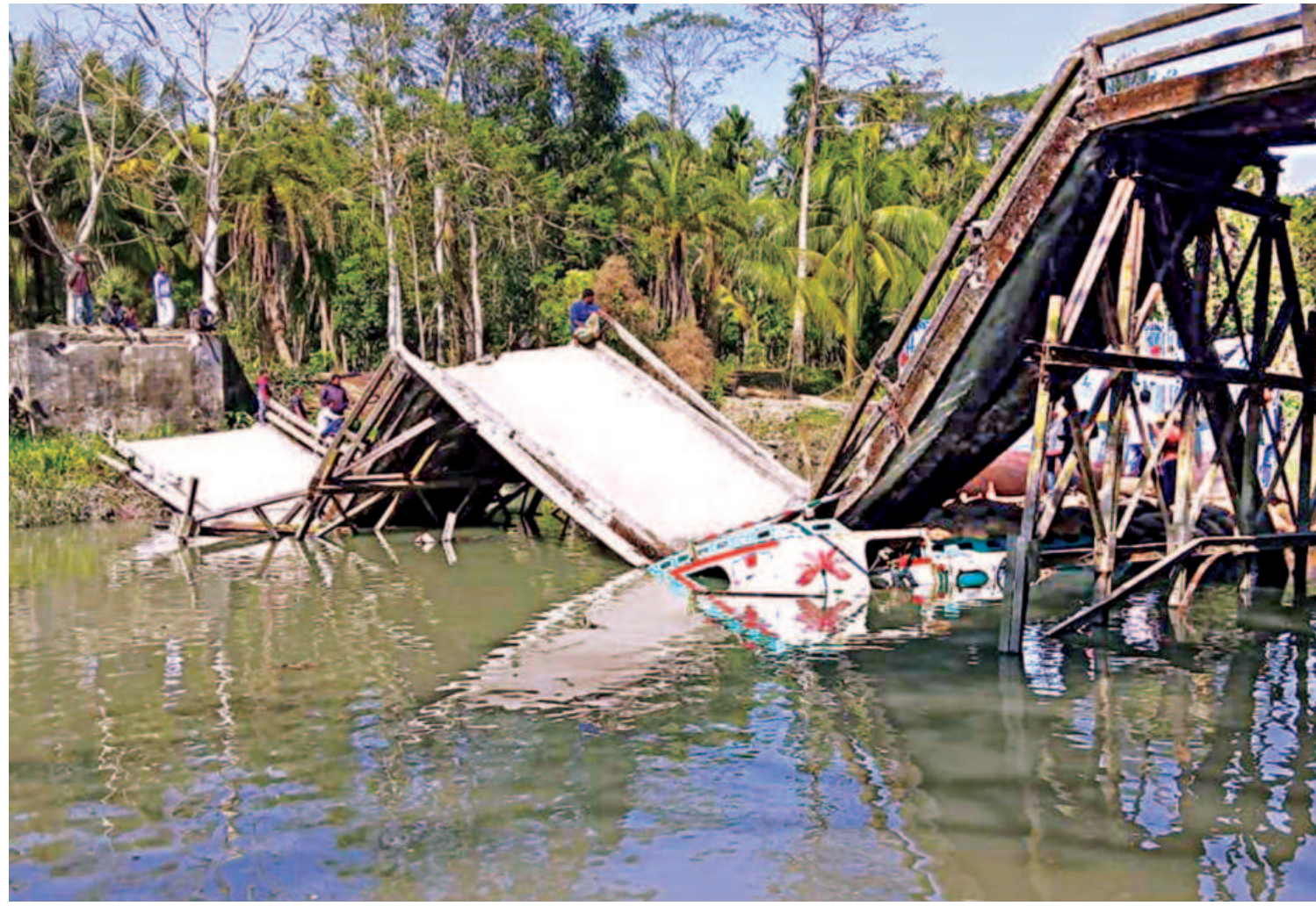
A sinking paddy-laden trawler that hit an iron bridge, causing it to collapse, in Domrabad-Hosnabad area of Patuakhali's Mirzaganj upazila on Tuesday. The accident has caused disruption to road communications between Patuakhali's Mirzaganj and Barguna's Betagi upazila and waterways communications between Jhalakathi and Khulna districts.
