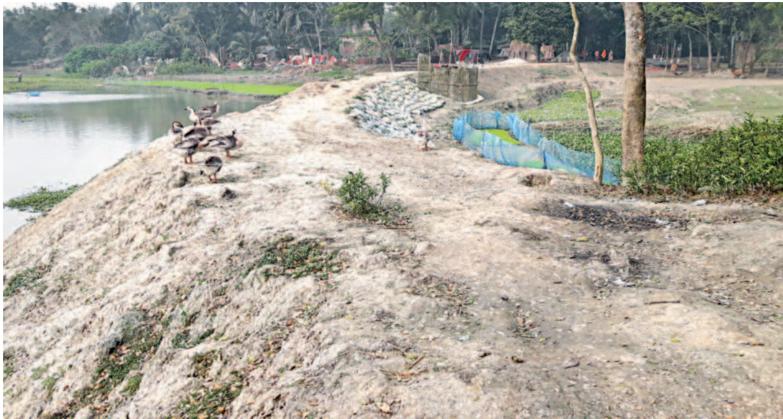
Embankment built at the mouth of Sonalidanga canal in Jhenidah's Kaliganj upazila impedes flowing down of water from the adjacent Majdia beel, eventually inundating a large area of croplands in the area.
