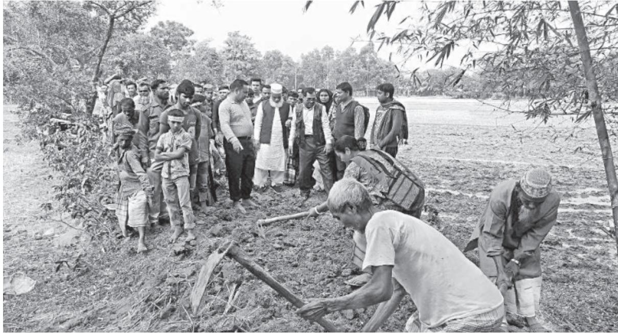
People of all ages join hands to repair this three kilometre road in Lengura union in Netrakona's Kalmakanda upazila yesterday. They took the initiative after repeated appeals to the authorities concerned fell on deaf ears.
