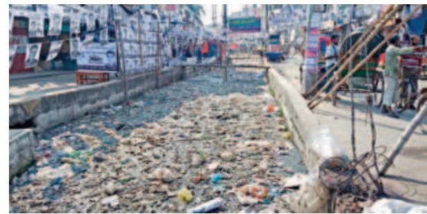
Kutubkhali canal filled up with waste.
