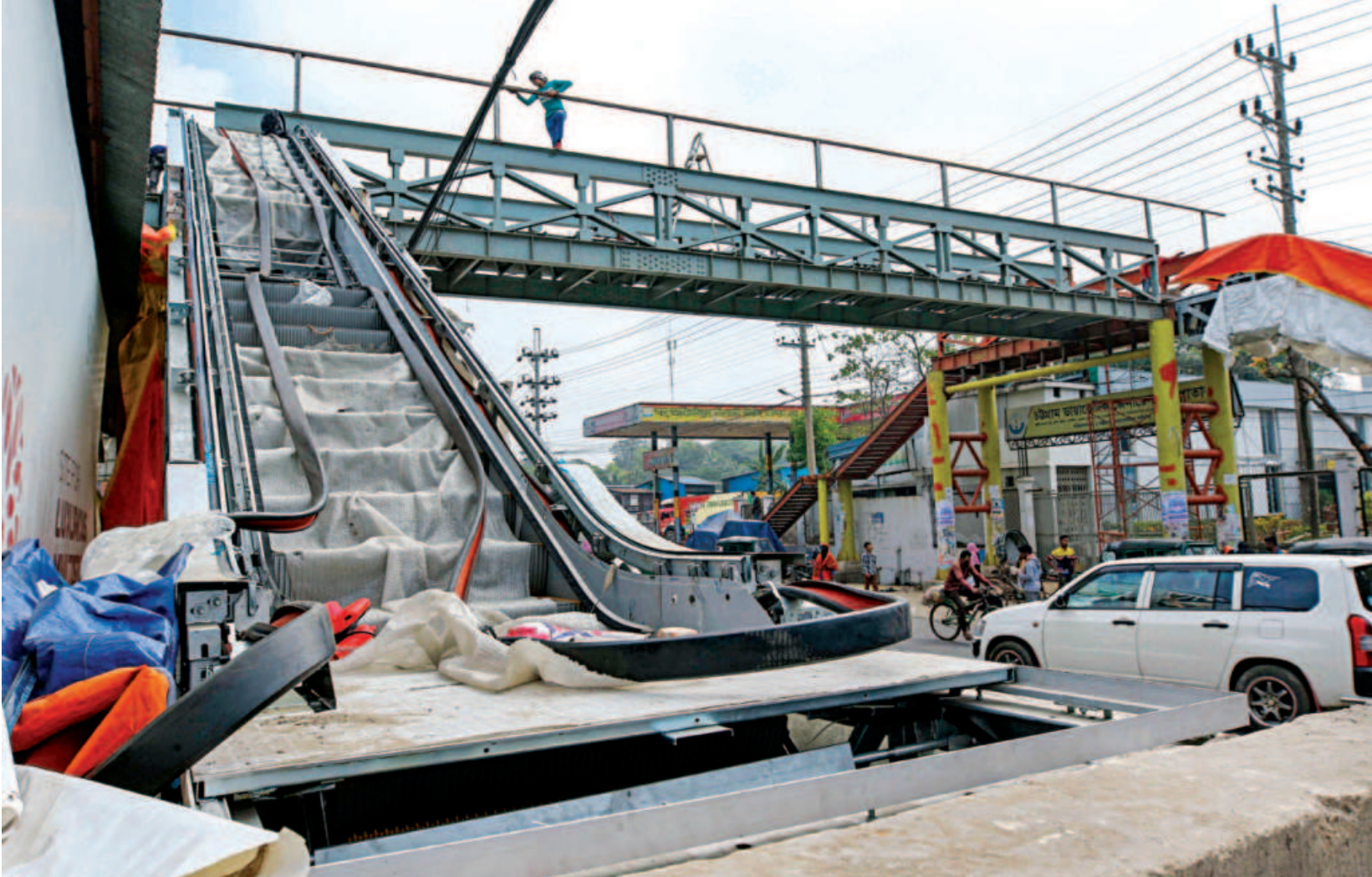
The Chattogram City Corporation installing escalators on a footbridge on Zakir Hossain road adjacent to Chattogram Diabetic General Hospital in Khulshi yesterday afternoon. This would be the first electric pedestrian escalator in the port city.
