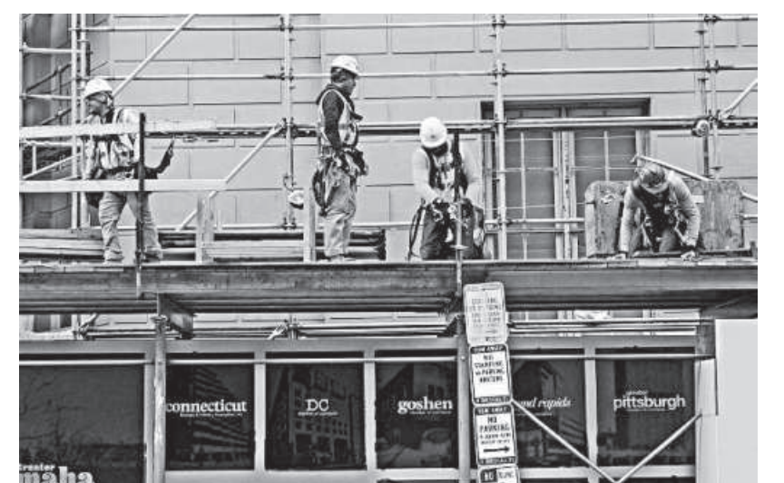
Construction workers put up support scaffolding on the side of a building in Washington.
