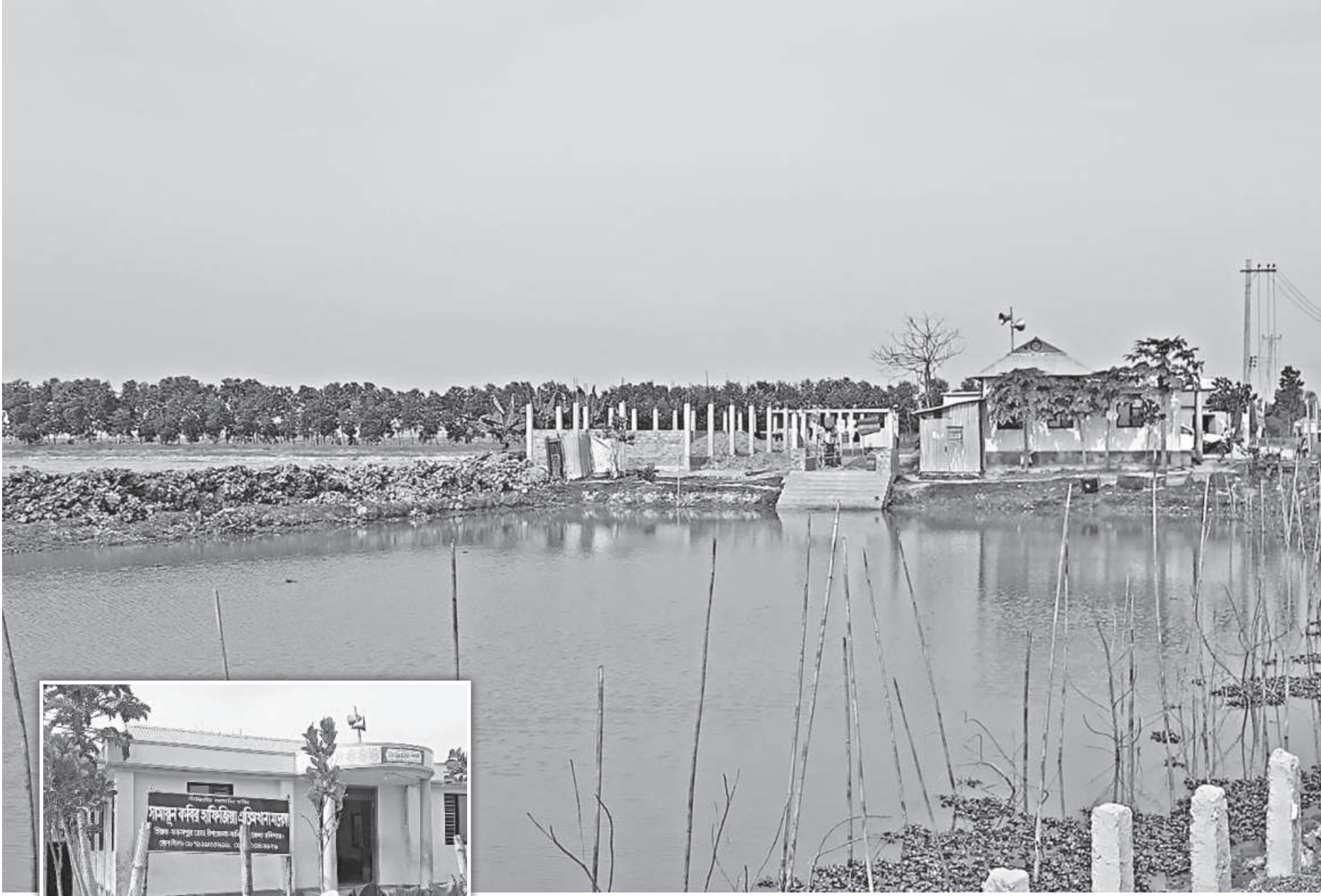
A land grabber has built illegal structures on the government land at Kachuarabda village in Habiganj's Baniachong upazila. Inset, a madrasa was built there by a local Krishak League leader.
