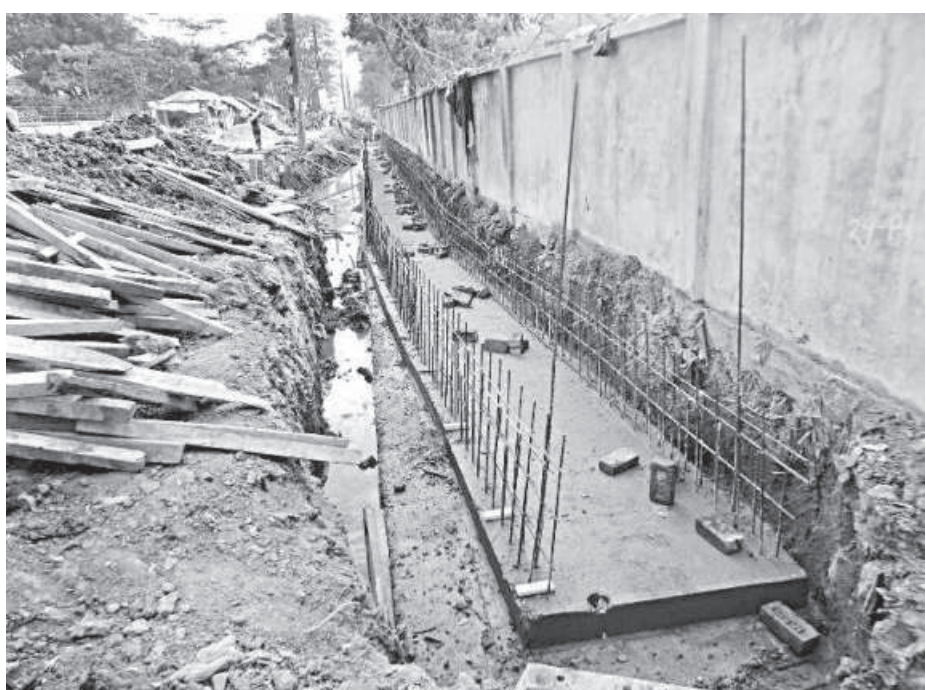
The under-construction drain along College Road in Patuakhali town.
