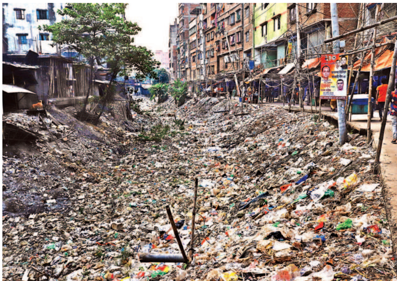
The Suvaddya canal is in its death throes as dumping of waste and rubbish into the canal goes on unabated. The photo was taken in Alam Market area of Dhaka's Keraniganj upazila recently.
