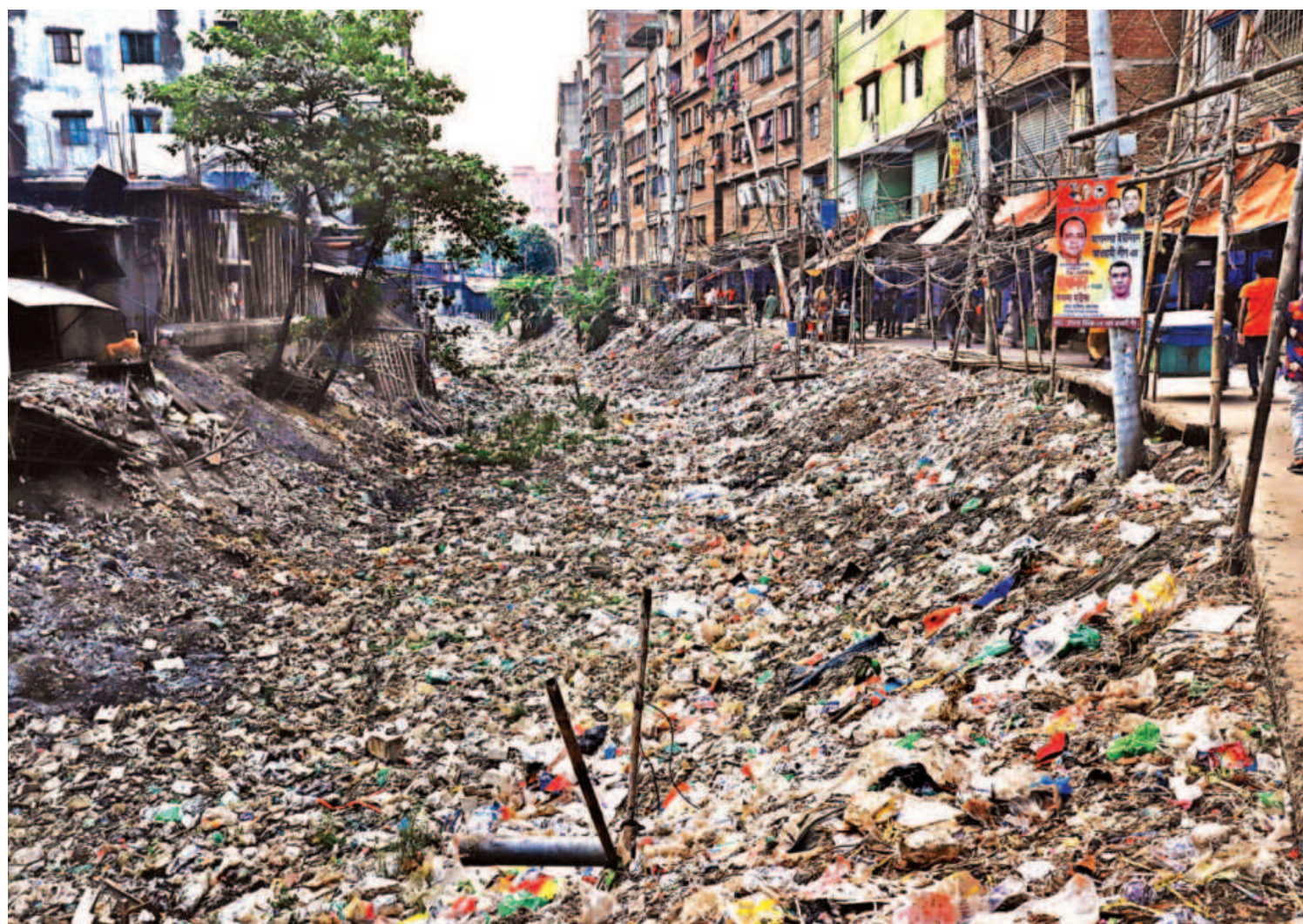
The Suvaddya canal is in its death throes as dumping of waste and rubbish into the canal goes on unabated. The photo was taken in Alam Market area of Dhaka's Keraniganj upazila recently.
