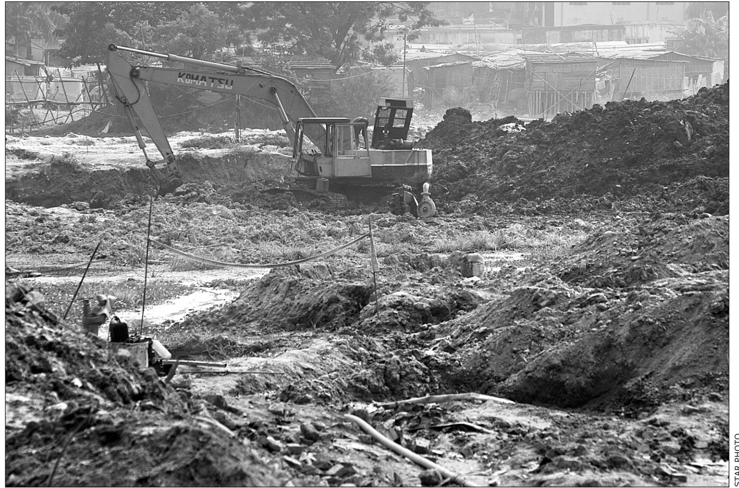
Work continues despite two notices served by Rajuk.
