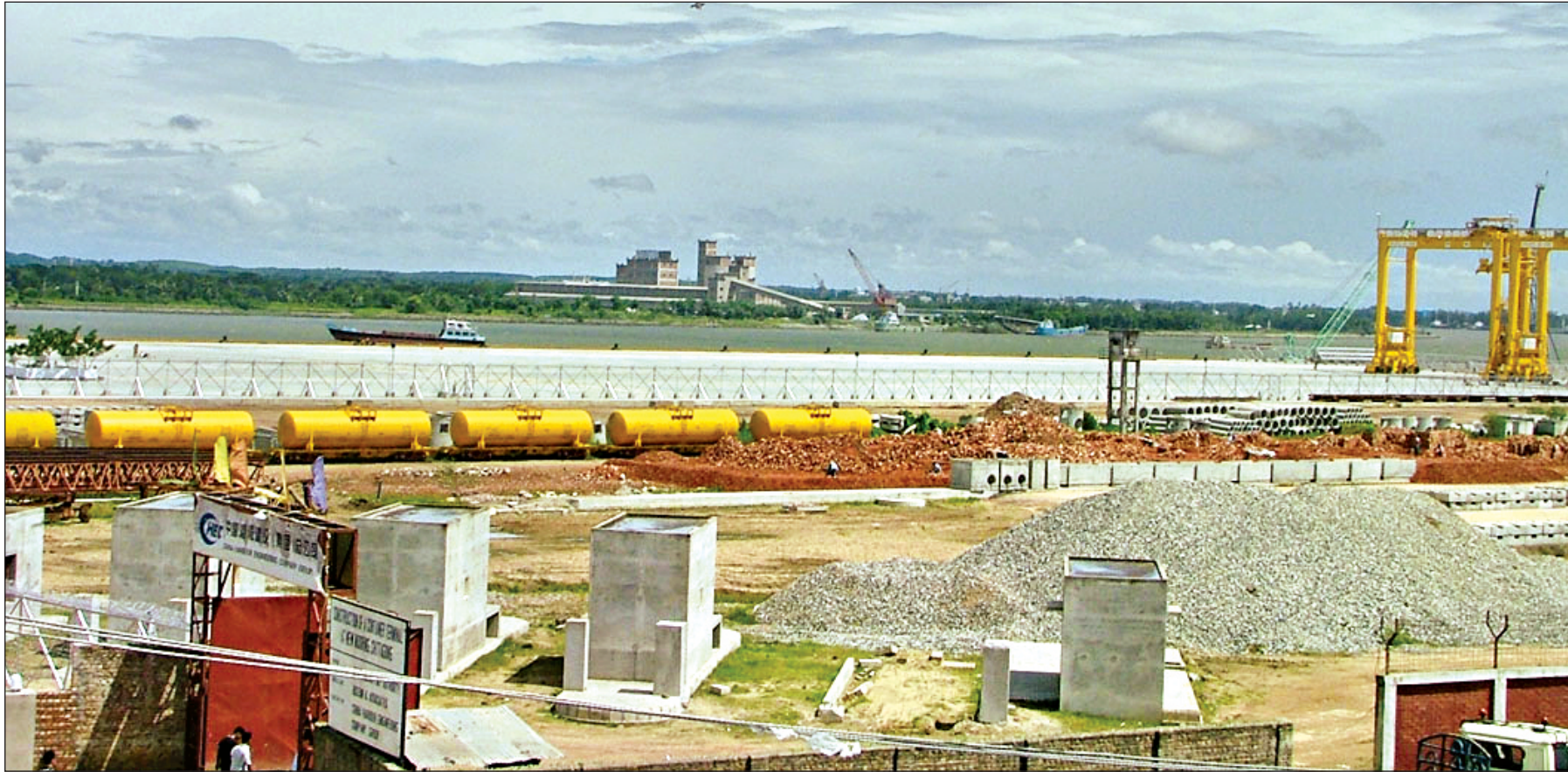
The under-construction New Mooring Container Terminal
