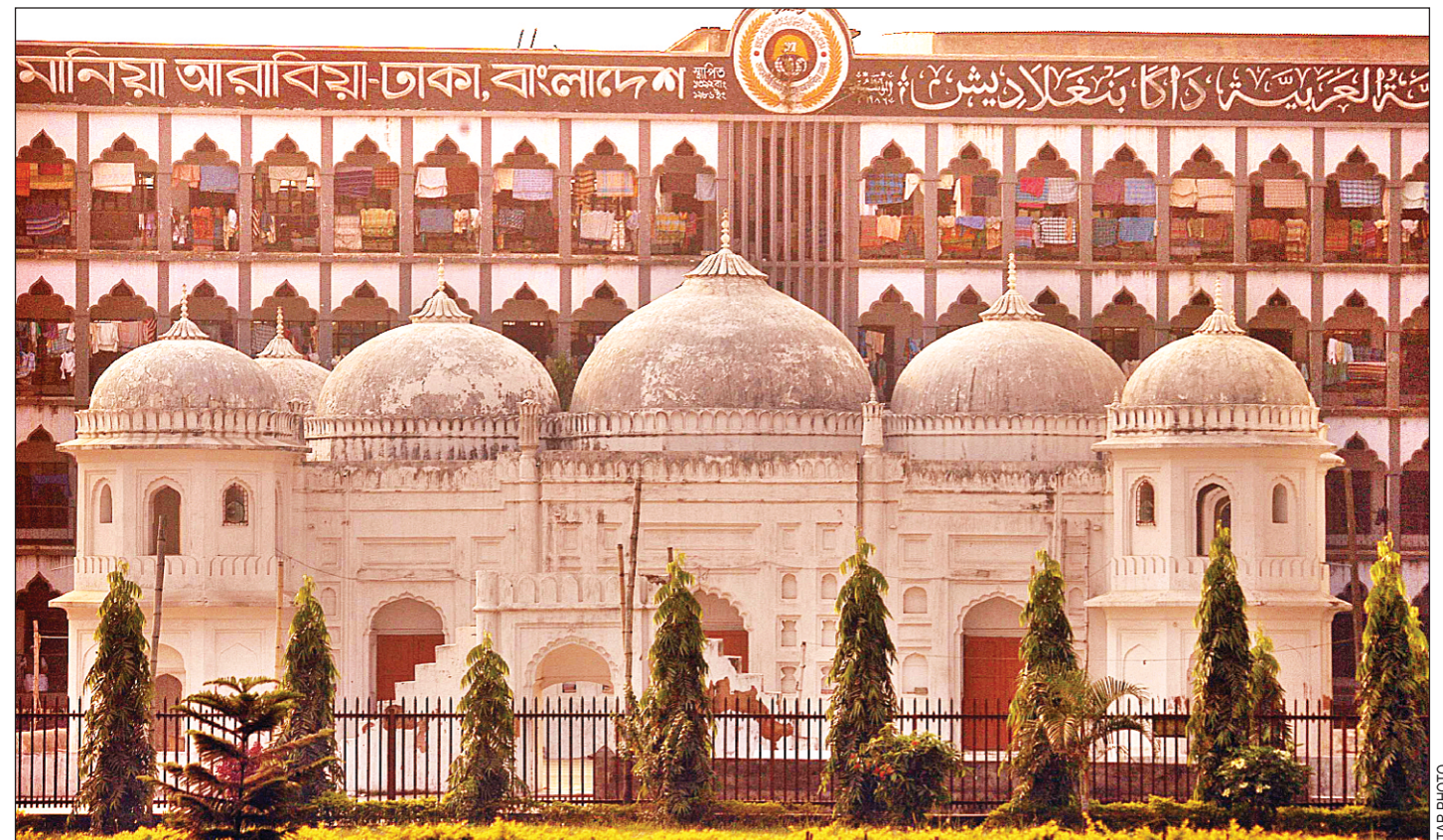
The historical Satmasjid in Mohammadpur area has been subjected to whitewash with its adjacent landscape spoilt by mindless construction.
