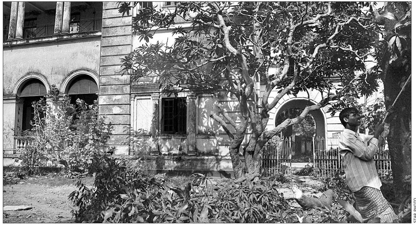
The 150 years old building of Jagannath University that faces total demolition.
