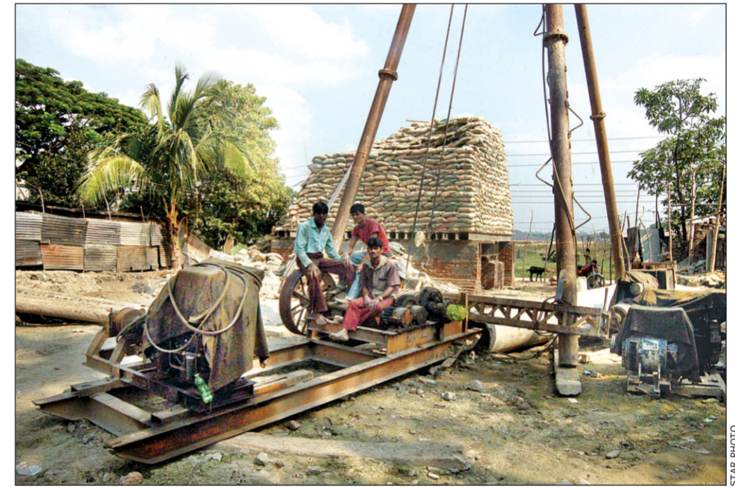
Construction of the third Buriganga bridge continues.
