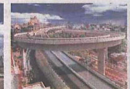
Khilgaon Flyover, Dhaka
