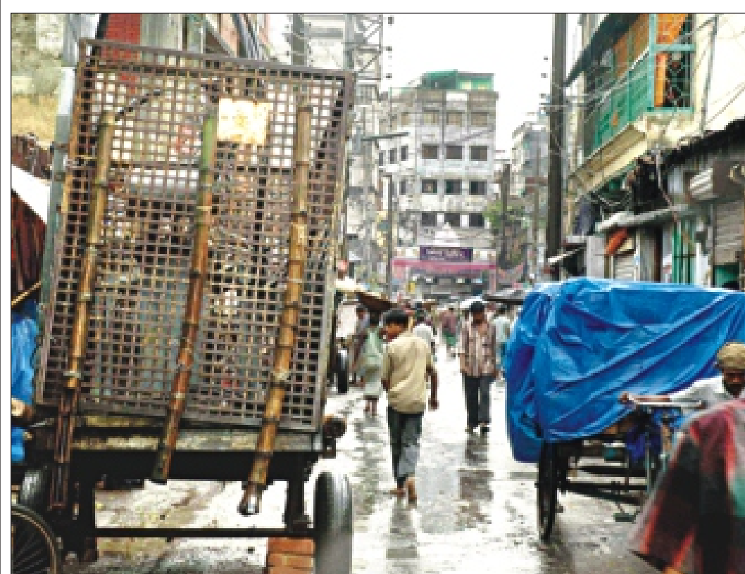
A power transformer placed inside a cage on a cart at Posta intersection of Laibagh in the capital. The transformer was installed there months ago obstructing movement of Old Dhaka residents on the narrow lane.
