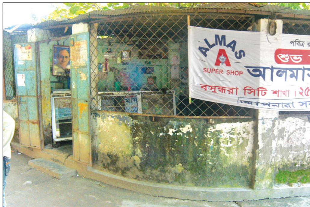
One of the illegal structures on the Abahani playground.
