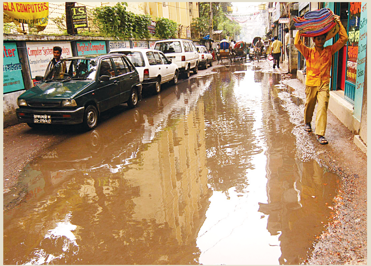
While the Nagar Bhaban keeps spending crores for renovating city's VIP roads the narrow street called Laboratory Road, off New Elephant Road remains waterlogged and dilapidated with large potholes. For over three months residents along this road have been suffering silently. Will our mayor please look into it?
