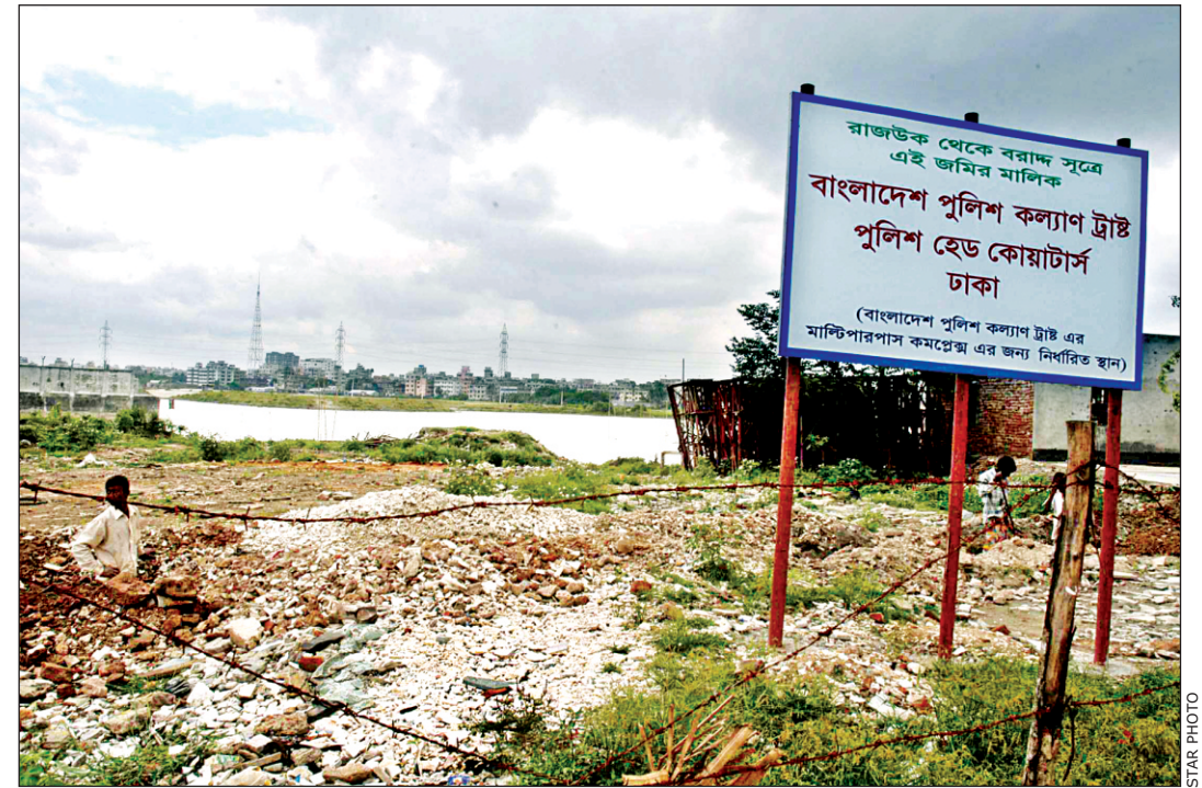
The housing ministry has handed over this Gulshan plot to police, where DCC is planning to construct a link road.
