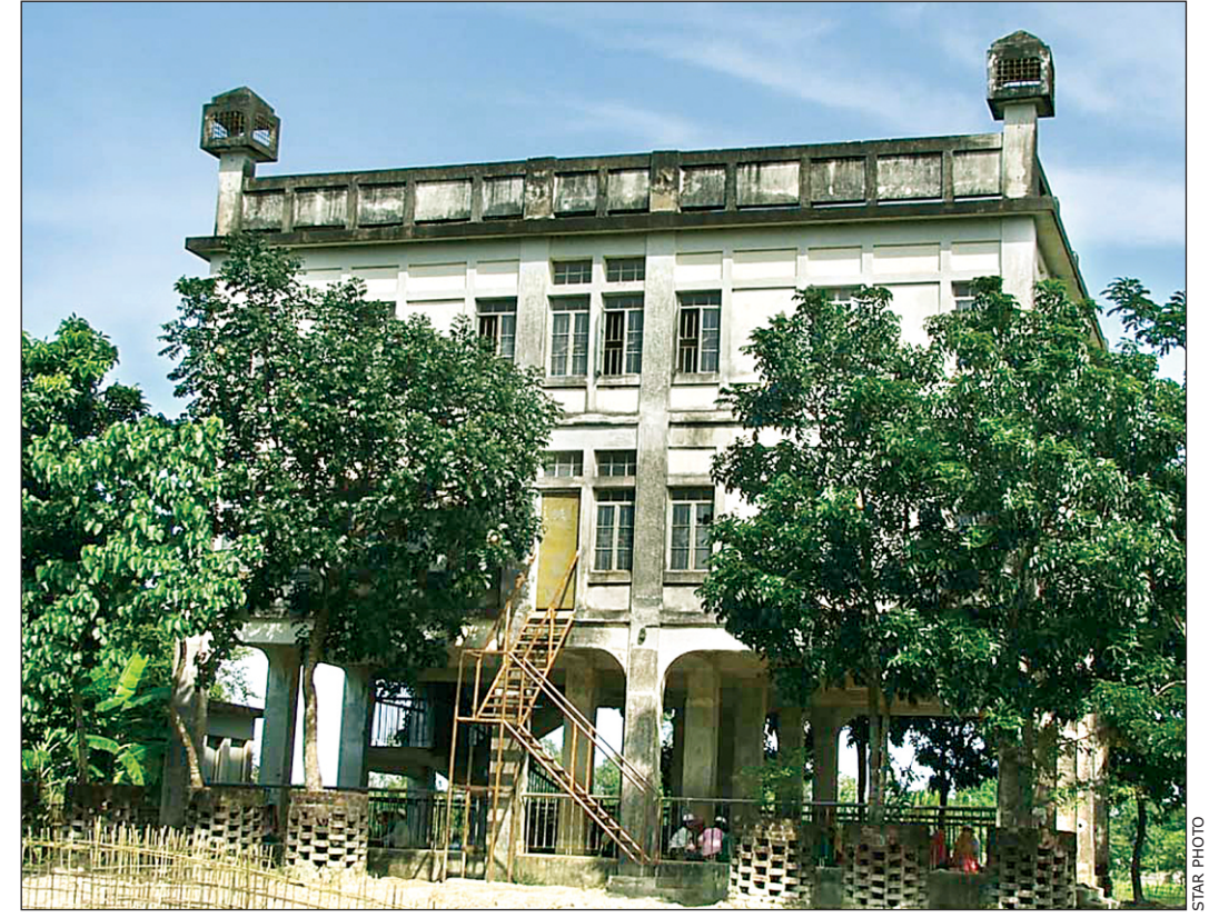
A cyclone shelter in Sitakunda.
