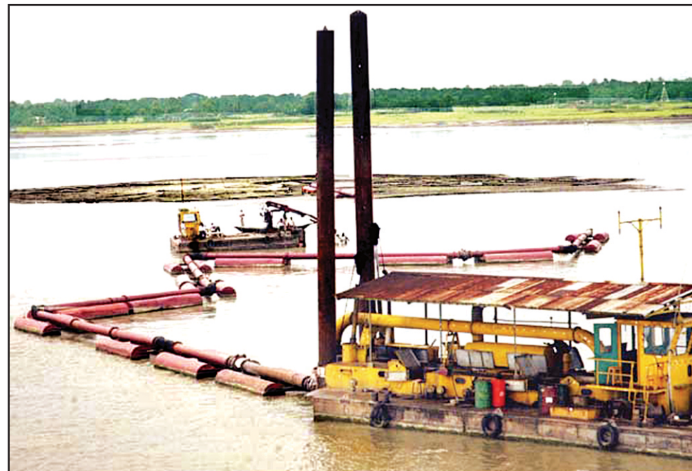
Dredging of Patria-Daulatdia channel in the Padma continues to make it navigable as the water level has fallen drastically in the monsoon (left) and a snarl-up of vehicles at Paturia ferry terminal.
