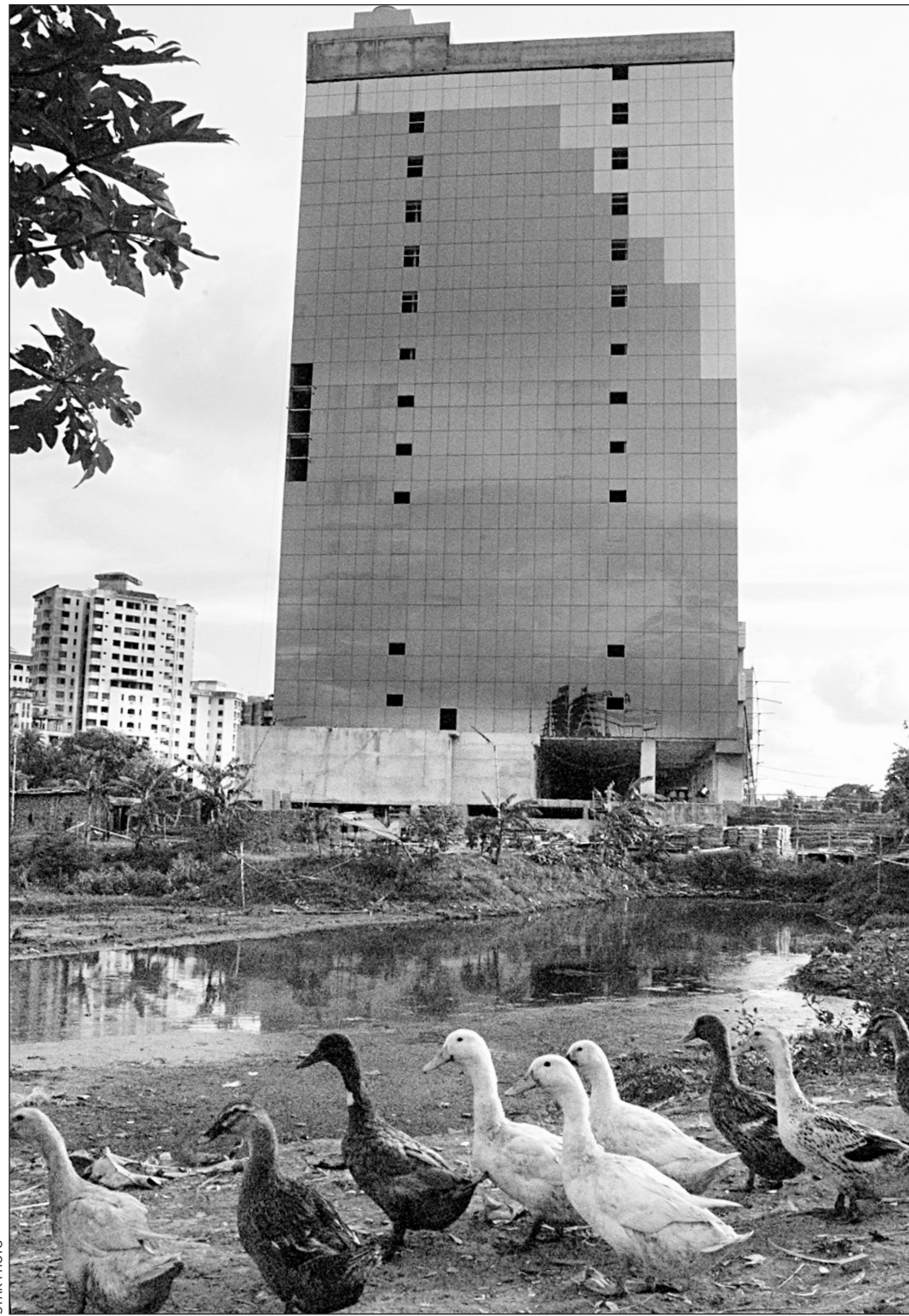
New BGMEA building under construction at Begunbari canal.
