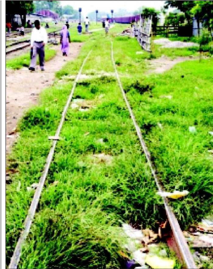
Uncared for railway track at the city's Tejgaon station. Long grasses have grown on the line and slum dwellers dump garbage at several points although trains run on it.
