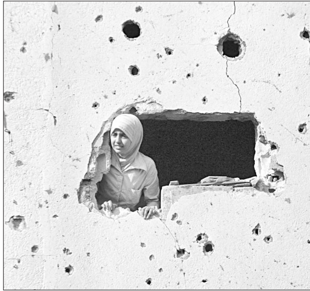
A young Lebanese woman looks from a hole in the wall of her building in the southern village of Saksakieh after it was hit by an Israeli air raid yesterday. Israel launched a wave of air strikes on southern Lebanon after issuing a new warning to residents to flee the area, which has repeatedly been bombed during the 10-day offensive.
