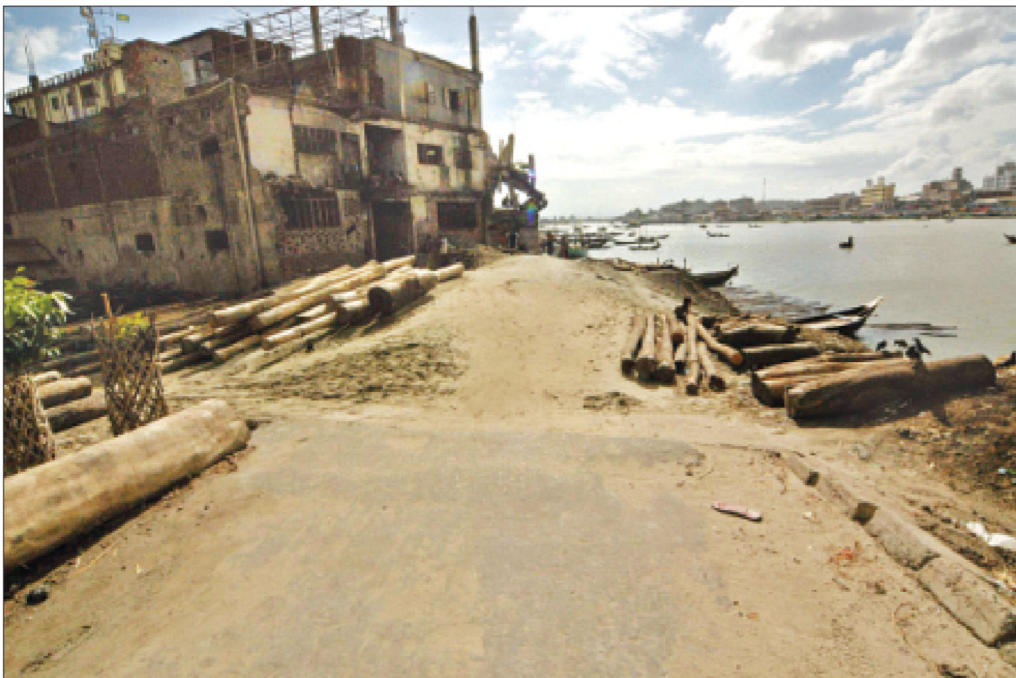
Illegally constructed just beside the Buriganga River, this building blocks the construction of a riverbank road by Bangladesh Inland Water Transport Authority.
