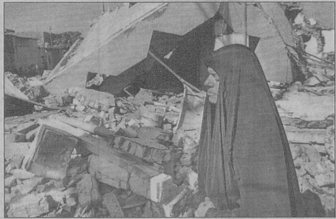
Wreckage of a house that was bombed in the restive city of Baquba yesterday, hours before the Iraqi prime minister unveiled a national peace plan.
